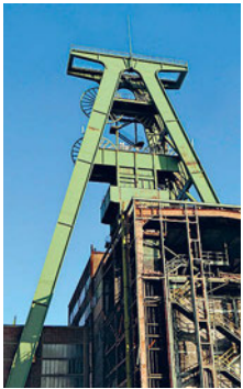
In 2020 RAG Aktiengesellschaft received the approval of the closure operations plan for the former Lohberg mine.
