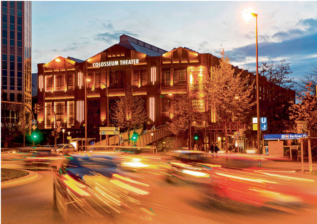
The listed Colosseum Theater in Essen: through the investment in this 120-year-old property, the RAG-Stiftung is actively contributing to the transformation of the Ruhr region.
